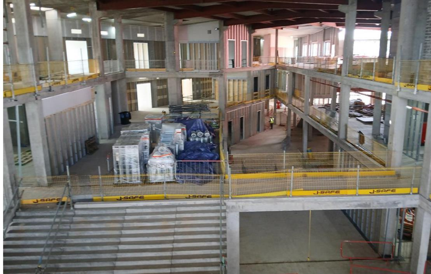
L2 Above Main Entrance Looking West
